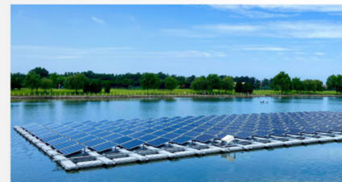
Floating solar system
