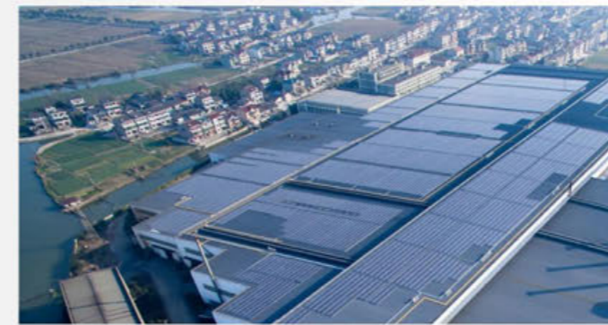
Commercial and Industrial solar system
